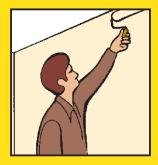
12.Apply 2nd coat of saturant (include seam)
